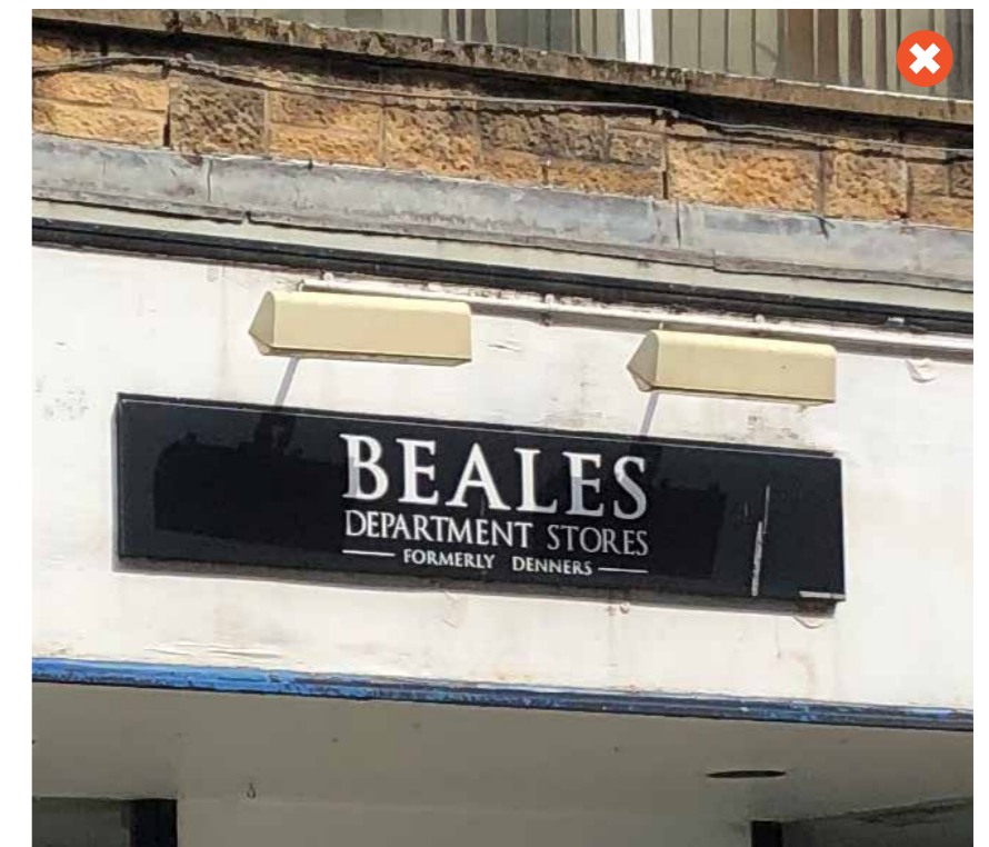
Figure 43. Lighting brackets too bulky and unattractive
