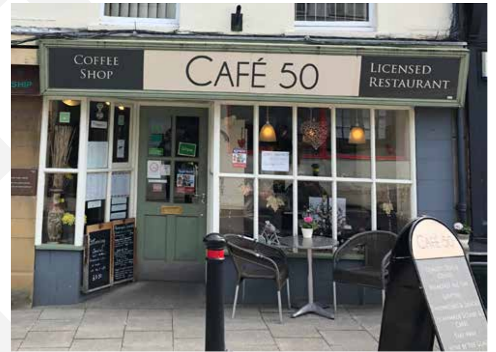
Figure 24. Recessed doorway and increased window display, door matches shopfront style
