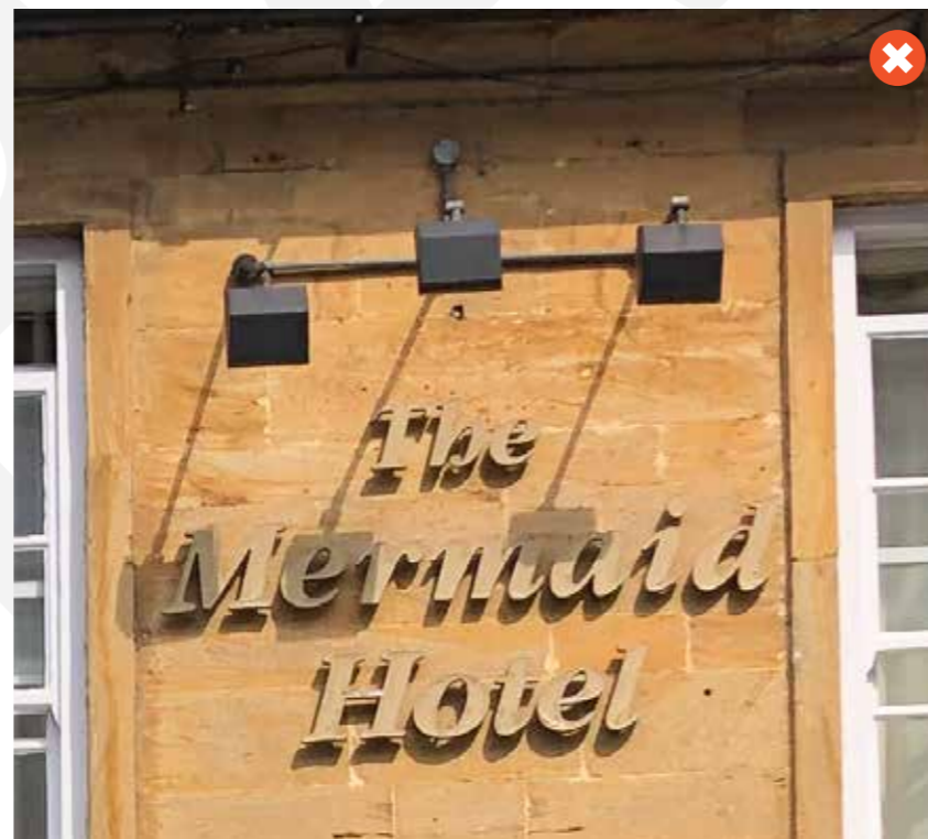
Figure 42. Lighting brackets misaligned and detract from building and sign
