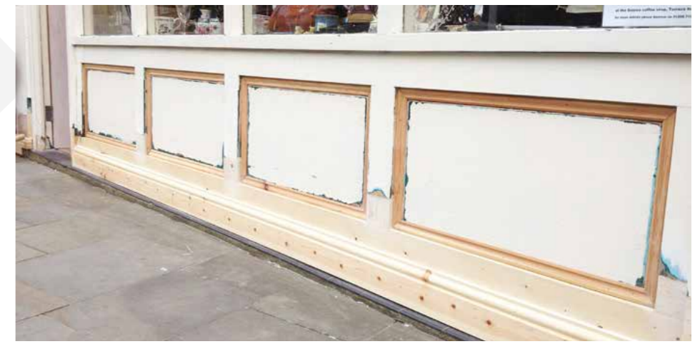
Figure 56. Timber stallriser repair
