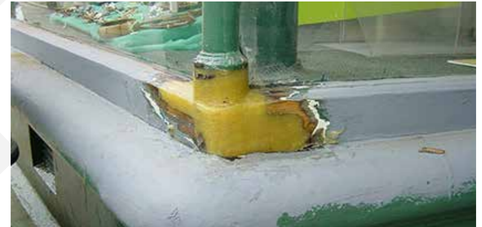
Figure 55. Resin repair to timber shopfront detail
