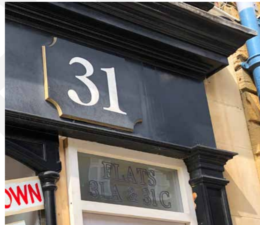
Figure 18. Projecting cornice, fascia and the capital topping the pilaster details respecting the building character – no console bracket.
