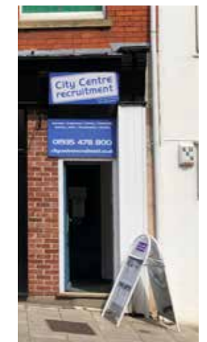
Figure 28. Signage disregards building elements
