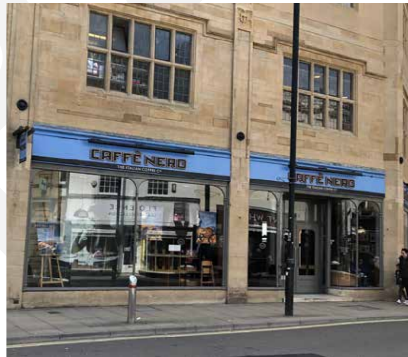
Figure 22. Contemporary shopfront in historic building designed to incorporate historic details
