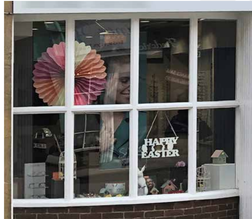
Figure 20. Timber mullions and transoms subdividing shopfront display
