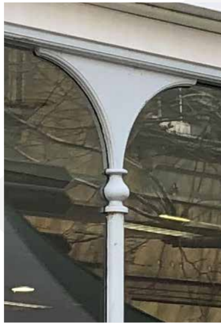
Painted timber mullion
