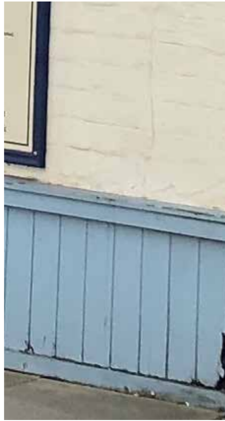
Painted brick and timber stallriser
