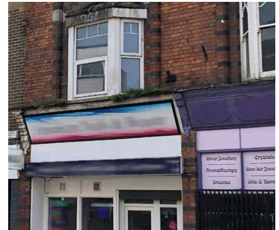
Figure 19. Console brackets allow fascias to be installed at an angle
