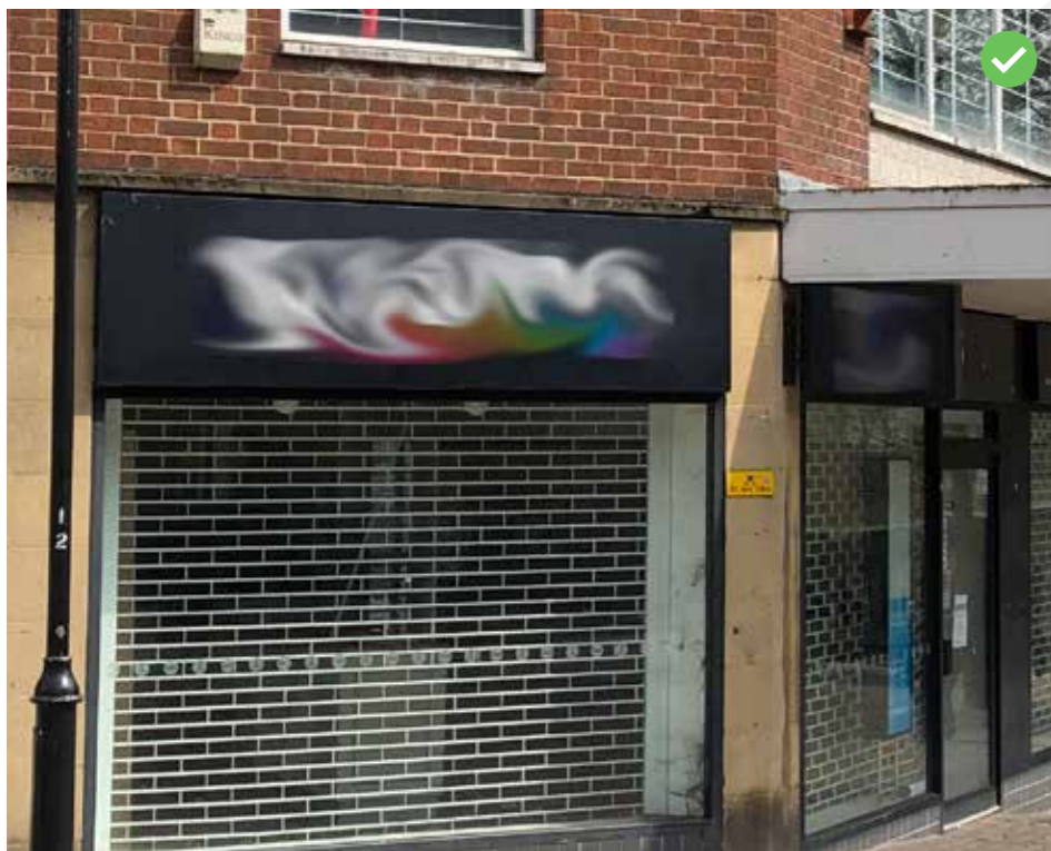
Figure 52. Open type, internal shutter integrated with shop type, generally acceptable
